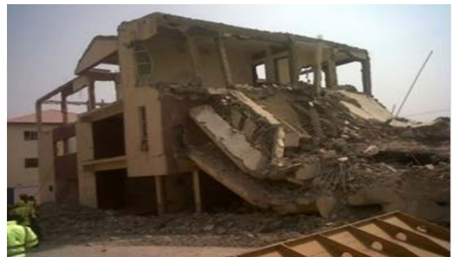
Plate 1: The Collapsed Naval Building located at Gwarimpa, Abuja, showing the wreckage. Source: Saharareporters, 2012)
