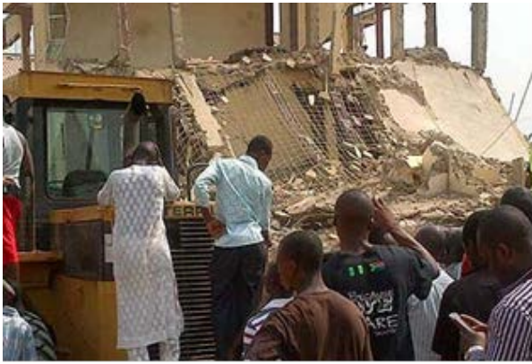
Plate 2: Clearing the debris on the Naval Building site (Source: Nnabugwu, 2012)
