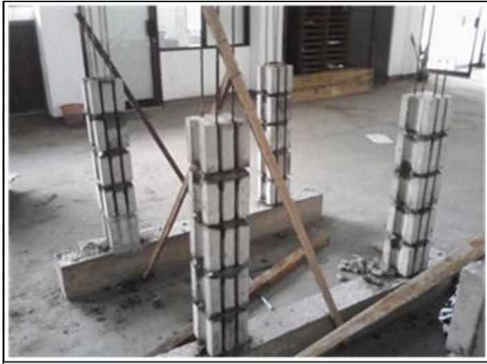
Figure 1. Frame construction of precast block-masonry unit column
