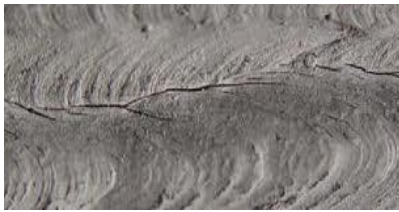
Fig. 2(a): Cold crack
