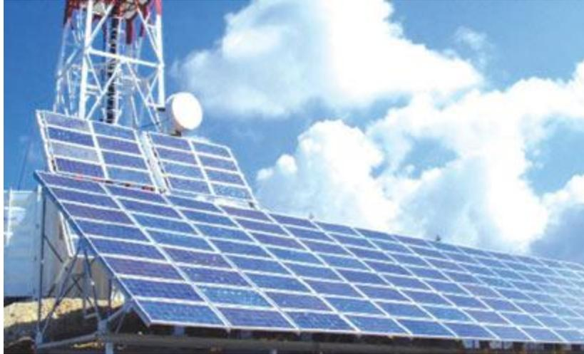
Fig 4: Photovoltaic cells (PV) at BTS sites: Source: (Vangurad, 2011)
