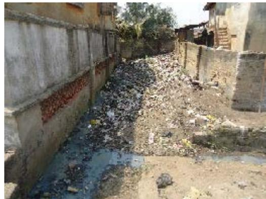
**Plate 3: Refuse dumped inside drainage channels which hinders free flow of run-off**
