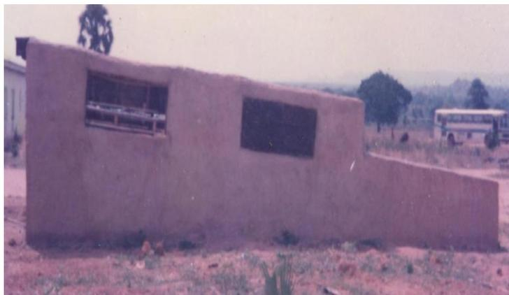
Figure 4: Solar dryer with mud solar thermal collector
