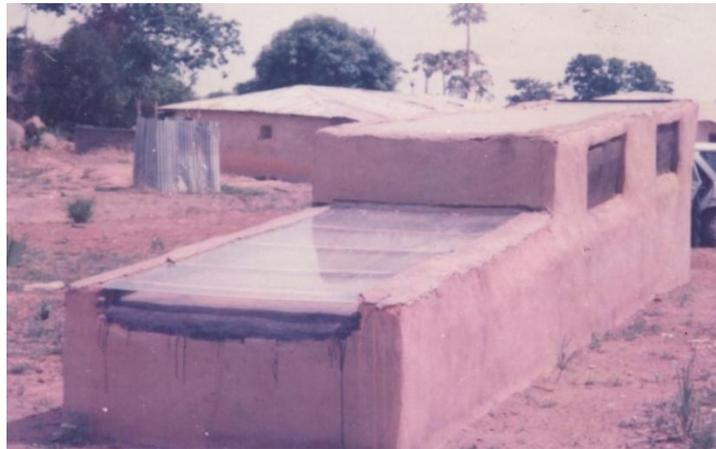
Figure 3: Solar dryer with cement solar thermal collector
