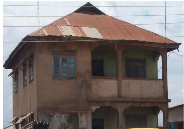
**Plate 8: A building along Arakale showing the flaking of paint and separation of layers**
