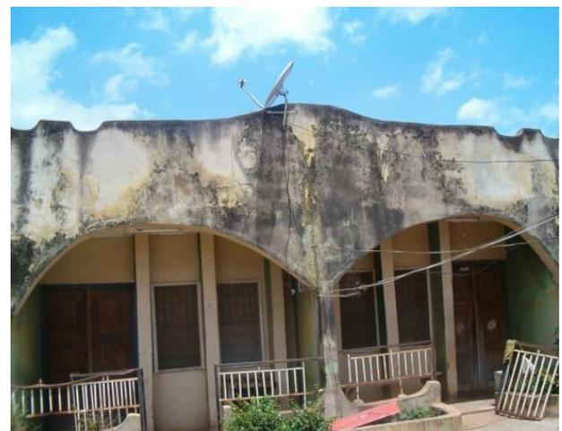
**Plate 9: A building along Arakale road showing physical weathering**
