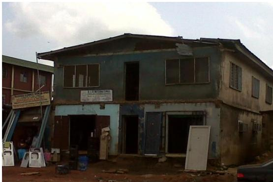
**Plate 11: A building along Arakale road showing discolouration of paint and dampness of the finish**
