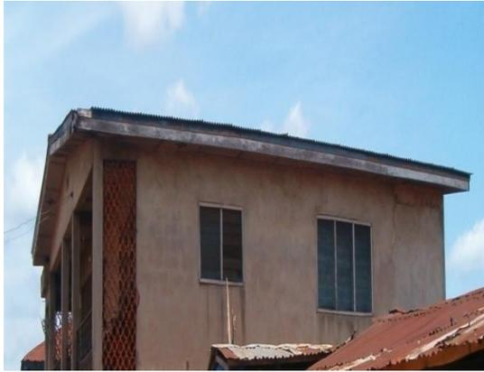
**Plate 10: A building along Arakale road showing dirt on the plastered surface**
