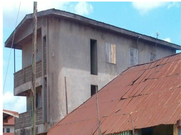
**Plate 6: A building along Arakale road showing microbial growth on the plaster finish**
