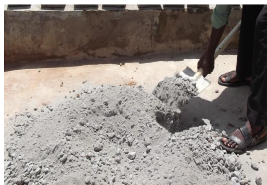
Plate 1b: Concrete Mixing on Concrete Platform
