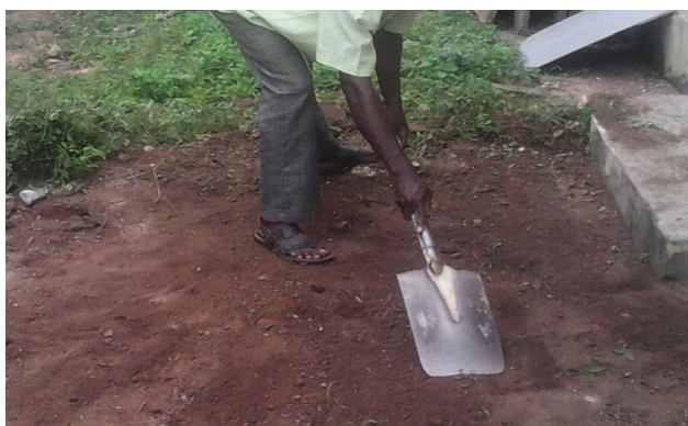
Plate 1a: Concrete Mixing on bare ground
