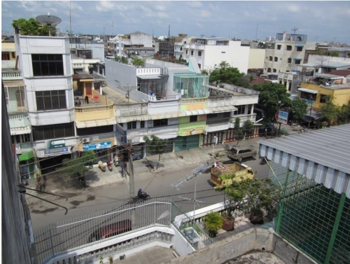
Figure 4. The density of buildings in Jalan Sutomo Ujung Medan
