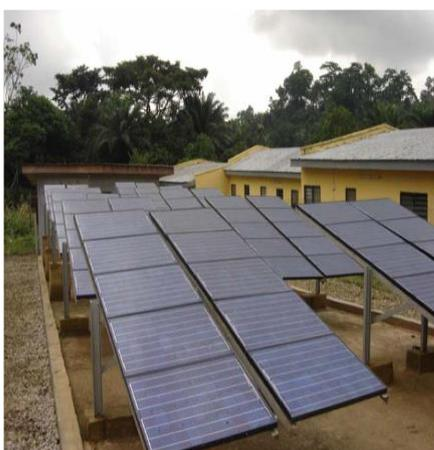
**Figure 1: Typical Photovoltaic Array Arrangement for the Investigated Water Pumping System**
