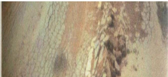
**Figure 1 Longitudinal cracks on a highway pavement at oniyale,ifo locality**
